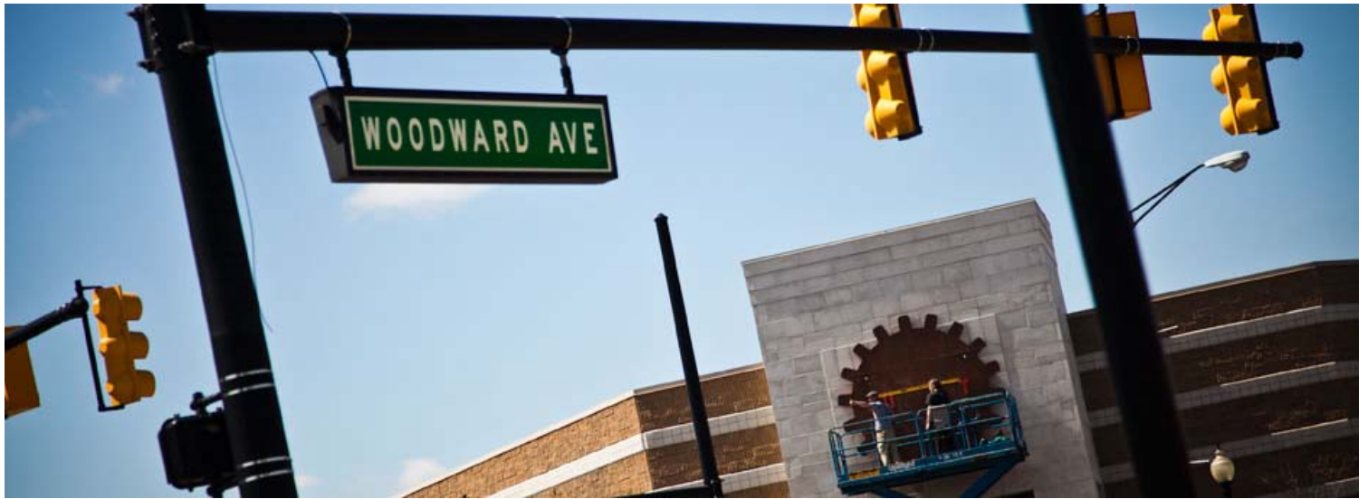
The Hanging of the Rustbelt Market Sign-Ferndale | David Lewinski
